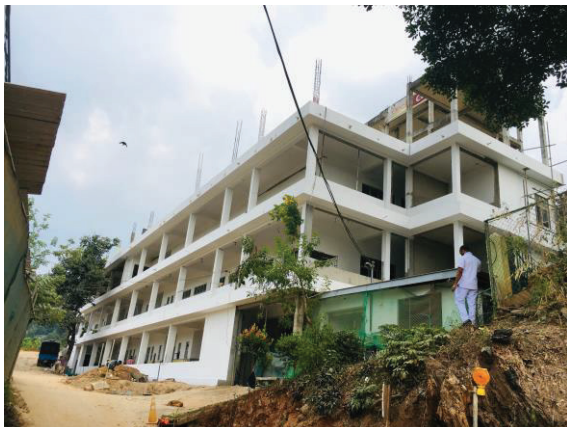
Isolation Building - Kandy
