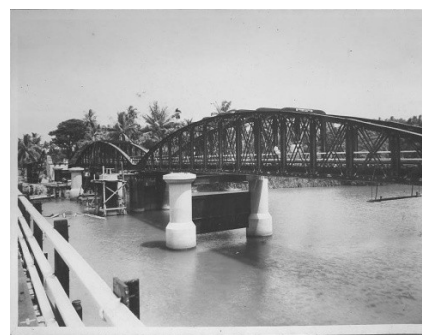
Thoppuwa Bridge 24 October 1938
