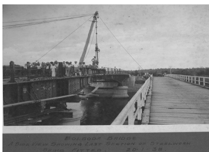
Bolgoda steel bridge –Side view
