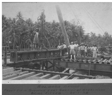
Bolgoda Bridge- Front View
