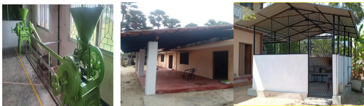
Fig 7: Maintenance and reconstruction work of production centers: Karainagar, Kattukkaran Housing Scheme, and Varothayanagar
