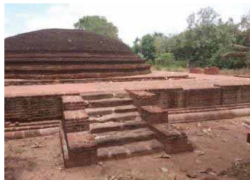
Conservation of the Enclosing Wall of the Meewalapathaha Stupa, Matale
