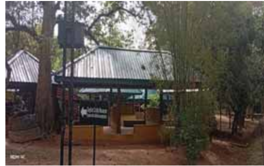
The condition of the stall roofs after they were repaired
