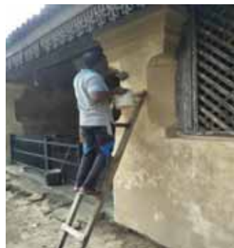
Maintenance of the Ambalangoda Dutch Stable
