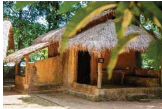
The condition of the ancient village cottages after renovation
