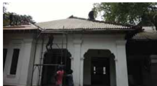
During the renovation of the roof of the office section of the Mahawalawwa Hall
