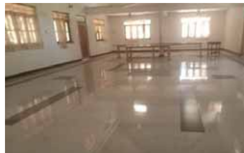
Completion of the remaining works of the Preaching Hall at Theraputtabhaya Raja Maha Vihara, Hambantota
