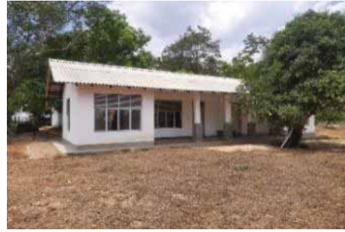
Completion of the remaining works of the official residence at Deegawapi, Ampara
