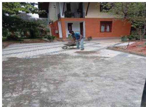
Applying floor tiles for new circuit bungalow at Anuradhapura
