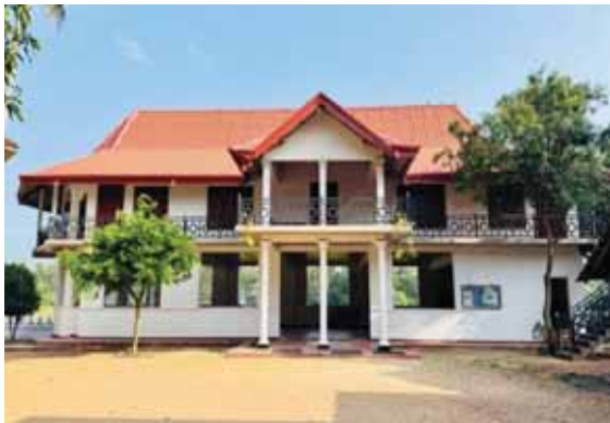
Completion of the remaining works of the Preaching Hall building at Sri Muni Gunarama Viharaya, Dankotuwa, Western Katukenda
