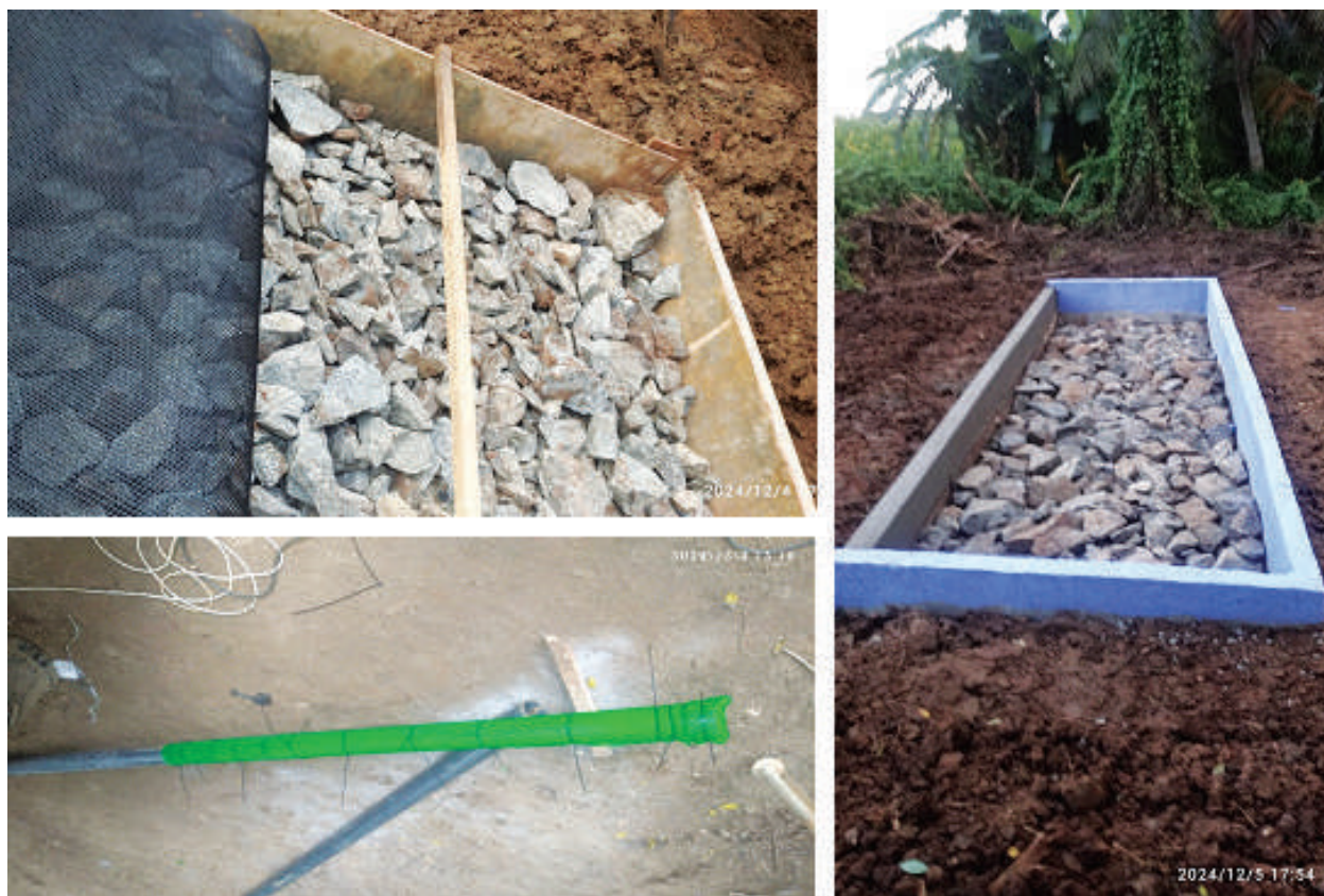
Figure 55 : : Final stage of the construction of Filter system
