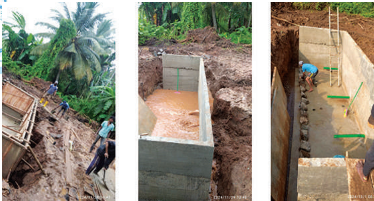
Figure 54 : Construction of recharge system (Filter system 1)
