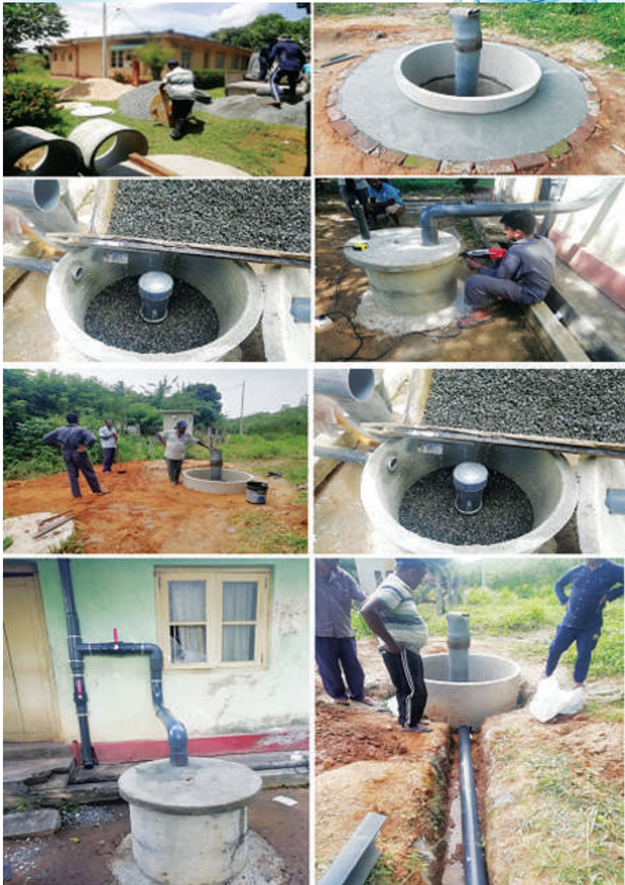
Figure 57: Construction of groundwater recharge system
