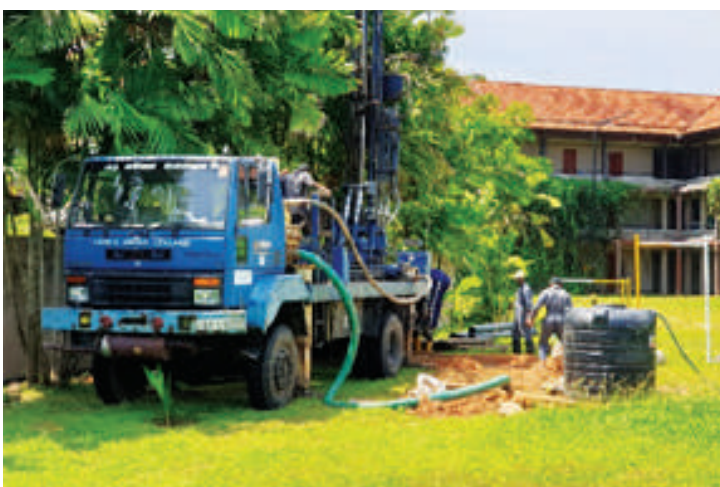
Figure 50: Construction of deep tube wells
