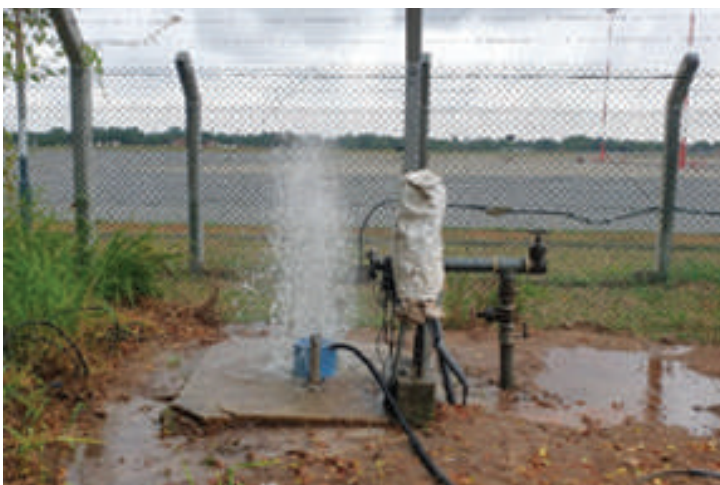
Figure 51: Tube well cleaning
