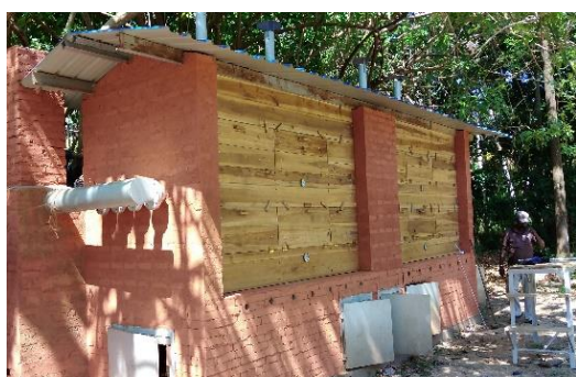
The dryer installed at the site
