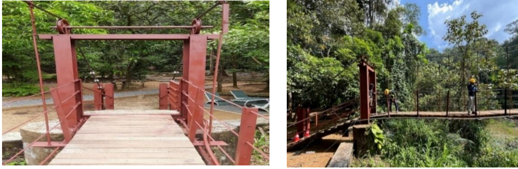
Figure 2.17 Renovation of the Pitadeniya access bridge of the Sinharaja Conservation Centre
