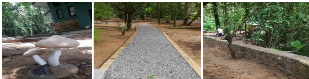
Figure 2.18: Improvement of landscaping
