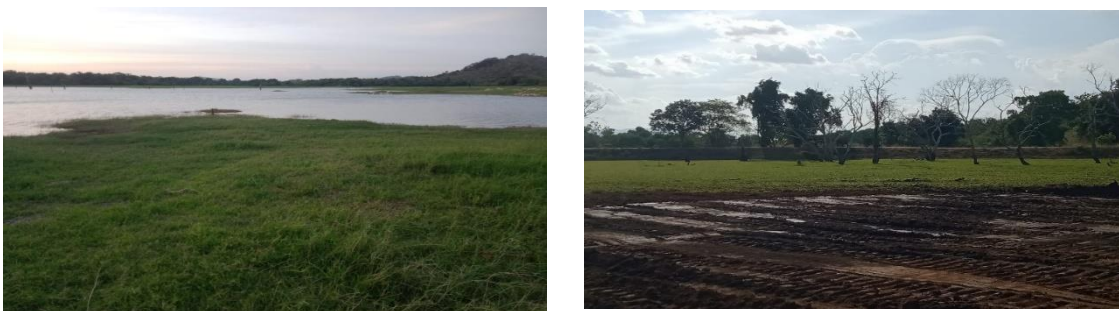
Figure 2.33: Removal of soil to increase the capacity of the Ihalakanda tank
