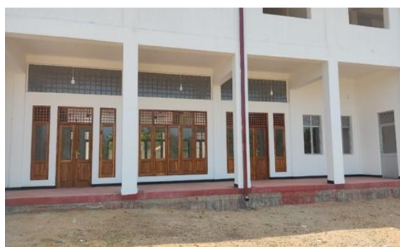
Construction of Vakaree New Court Building
