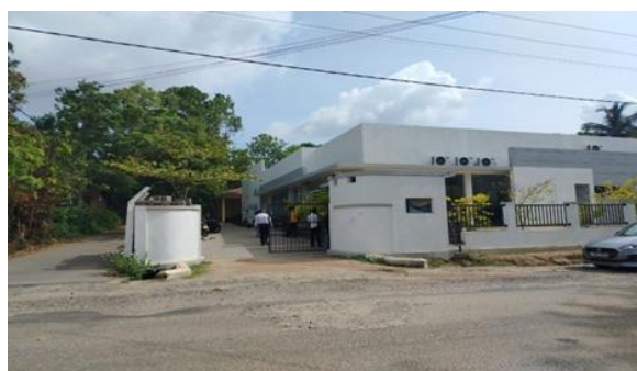
Construction of Nikaweratiya Prefabricated Court Building
