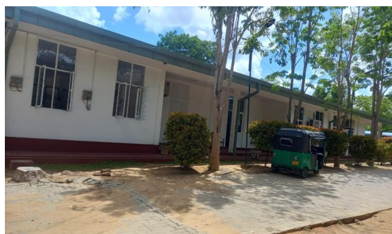
Construction of Samanthurai Prefabricated Court Building
