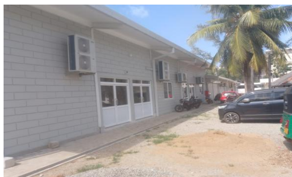
Construction of Puttalam Prefabricated Court Building
