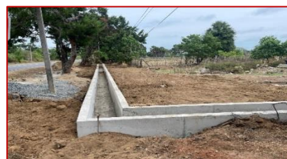
Drainage Construction - Kariyalaingapaduwan.
