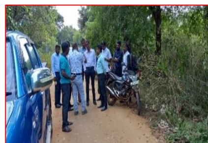
Field visit to monitor the renovation of Kiranji - Ponnaveli Road
