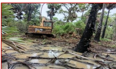
Deepening and Widening of Netheli river, 4 km stretch.
