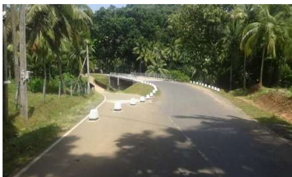
5125 + 5126, Dodangaslanda Katupilagolla Bridge in Kurunegala
