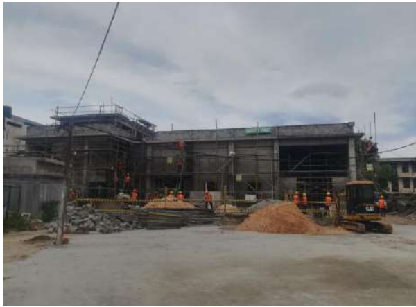
Kalinga Mawatha Pumping Station
