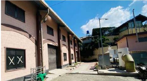
Thimbirigasyaya Pump station
