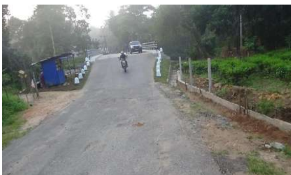
Bridge No 5172, Menerigama Bridge in Kalutara
