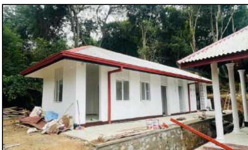
Constructions relating to Medadumbara Mihidan Uyana Project
