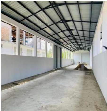
Project on construction of Material Recovery Facility in the Kattankudy Urban Council
