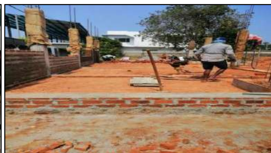
Constructions relating to the project of vehicle Park, Fitness and Sports store and corner at the Sri Albert F. Peris Stadium
