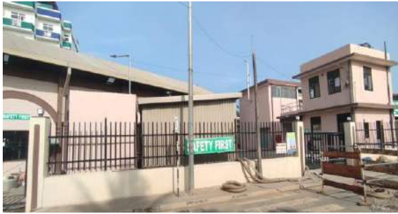
Vystwyke Pump station
