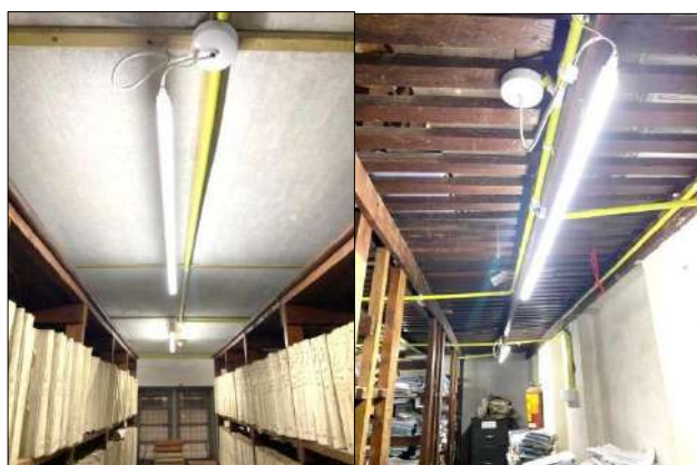
Rehabilitation of the Electrical System in the Record Room of the Negombo Land Registry
