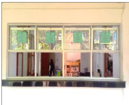
Renovation and Repair of Windows at the Avissawella Land Registry Office
