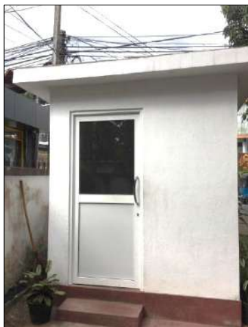
Security Guard Post at the Gampola Land Registry Office
