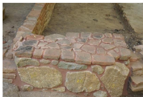
After conservation of the outer boundary wall no.3
