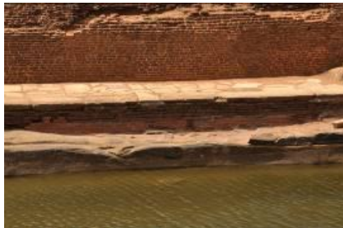
After conservation of walls around the Girikula Eastern Pond
