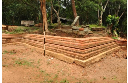
Before the conservation of Vijayarama Eastern Boundary Wall
