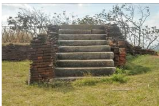
Before conservation of a staircase on the rock
