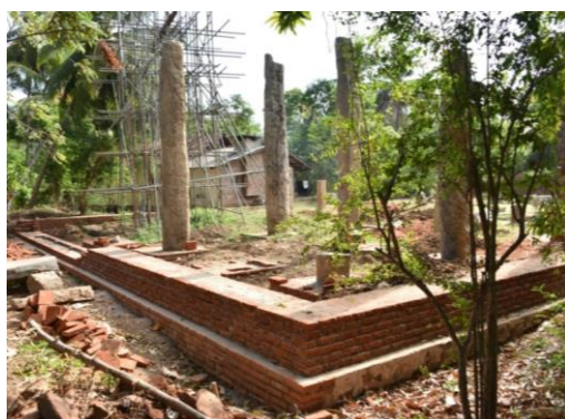
Before conservation of the Western Boundary Wall
