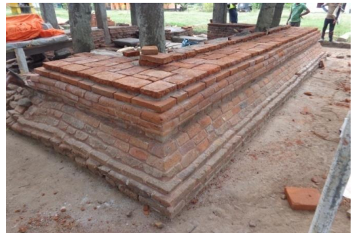
During the conservation of Mahatalakolawewa Image House
