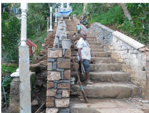
During conservation of the old staircase and railing walls of Vilwala Rajamaha Vihara
