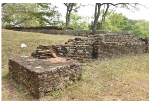
Before commencing scientific maintenance of the Outer Boundary Wall
