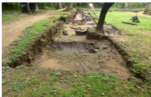
Before conservation of the Boundary Wall of Shiva Temple No.2
