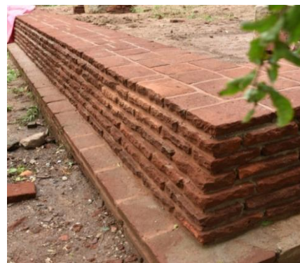
After conservation of the Western Boundary Wall
