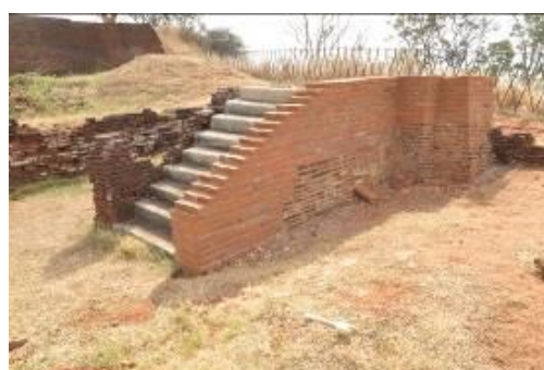
After conservation of a staircase on the rock
