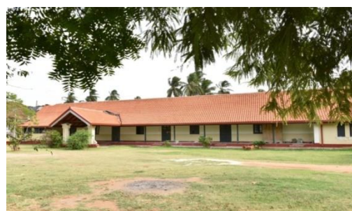
After conservation of the roof of the Tissa Vihara Hermitage
