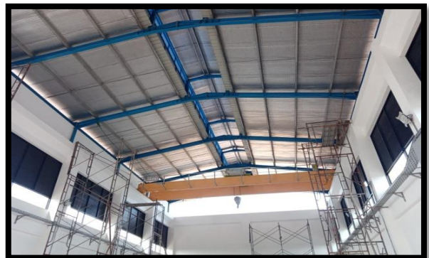
Figure 4: Installation of EOT Crane
