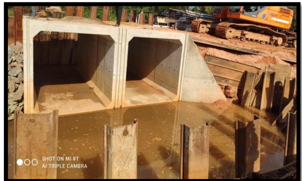
Figure 5: Construction of Box Culvert
