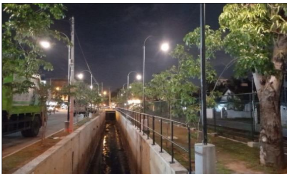
2.1-1 Concrete Canal Total Concrete Canal Length – Approx. 2.5 km
