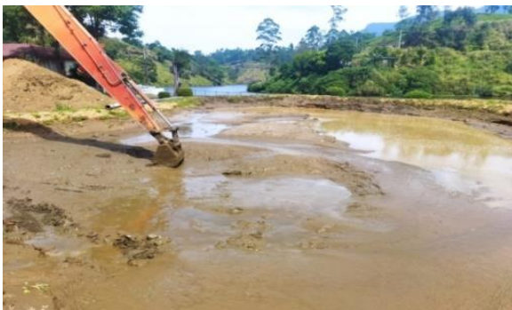
Figure 05: Progress of De- silting
