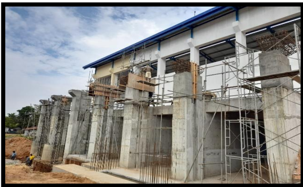
Figure 1: Construction works of Pumping Station II in January 2023
