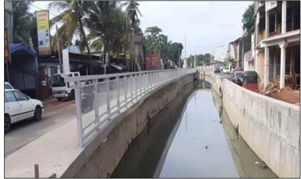
2.1-2 Sheet Pile Concrete Canal Total Canal Length – Approx. 0.5 km
