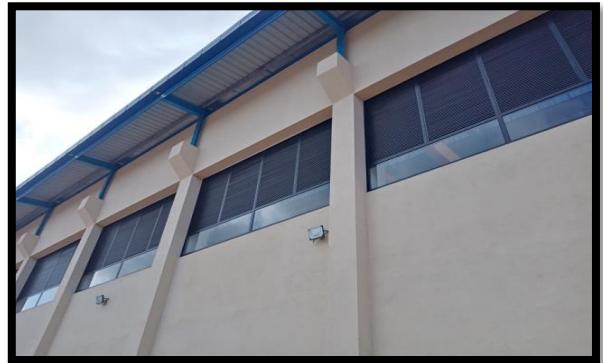
Figure 3: Installation of Aluminium Louvers and Roller Doors
