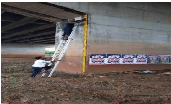
Figure 07: Installation of water level gauges
