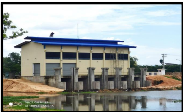
Figure 2: Construction works of Pumping Station II in December 2023
