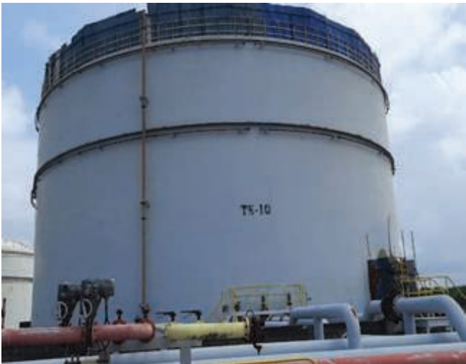
Proposed Tank No. 09 and Tank No. 10 for IFR Installation
