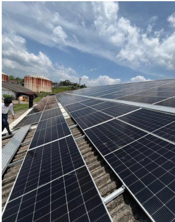
Installation of 300 kWp rooftop solar photovoltaic (PV) power generation system at Kolonnawa Installation
