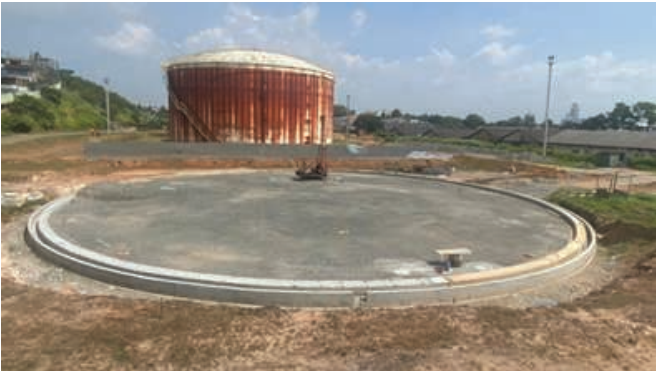
Construction of foundations of Tank B and Tank D at Kolonnawa Installation
