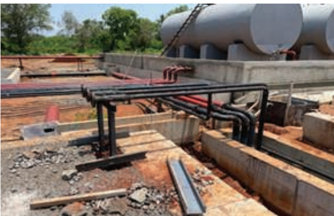
Construction of Tank Farm
