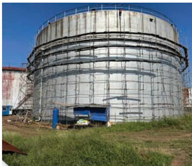
Repair work is in progress for Tank No. 21
