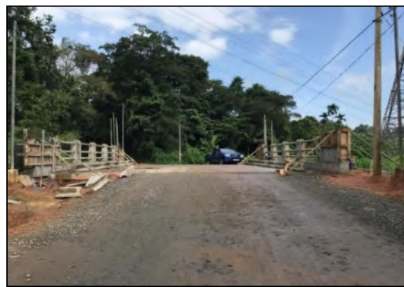
Figure 2-5: Design & Construction Supervision of Godigamuwa Bridge in Non-RDA Road.
