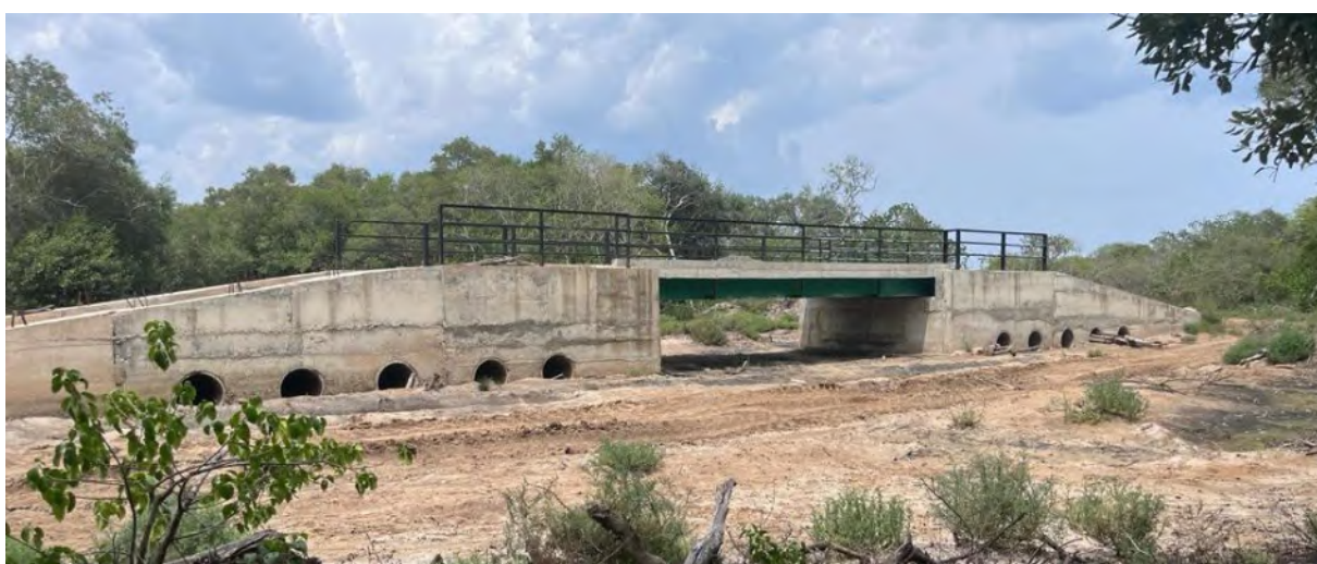
Figure 2-2: Construction of Bridge across Kokumodai aru on Thennamarawadi, Kokkuthuduwai Road at Kokumodai Mullaitivu
