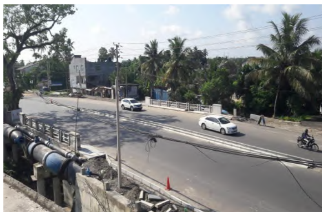
Figure 2-41: Completion of Bridge No. 6/2
