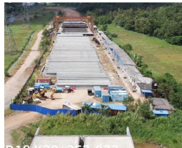
Figure 2-35: Ongoing work of CEP -I
