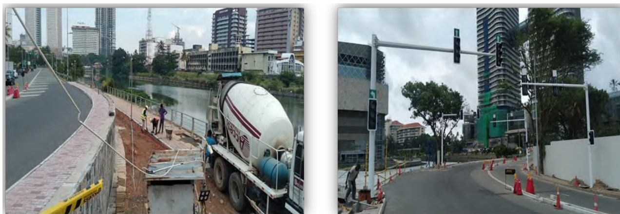
Figure 2-33: Flyover at Baladaksha Mawatha
