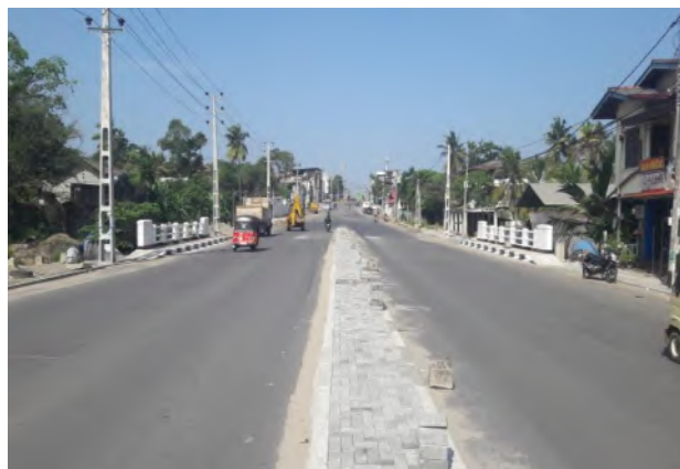
Figure 2-39: Completion of Bridge No. 6/1
