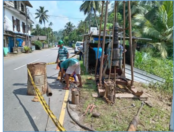
Figure 2-8: Borehole Investigation of Bridge. No- 22/5Km on Ambalangoda – Elpitiya –Pitigala Road
