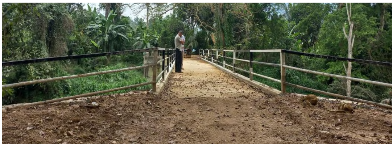
Figure 2-1: Construction Balance work of Bridge across Loggaloya at Thaldena Meegahakiula in Badulla
