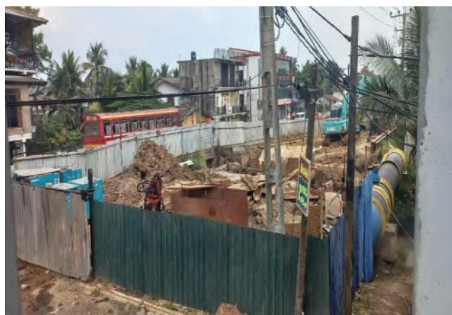
Figure 2-43: Widening and reconstruction of the bridge No. 4/2
