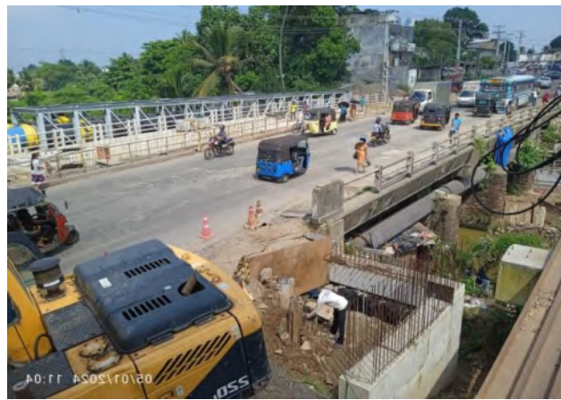
Figure 2-42: Widening and reconstruction of the Bridge No. 3/1
