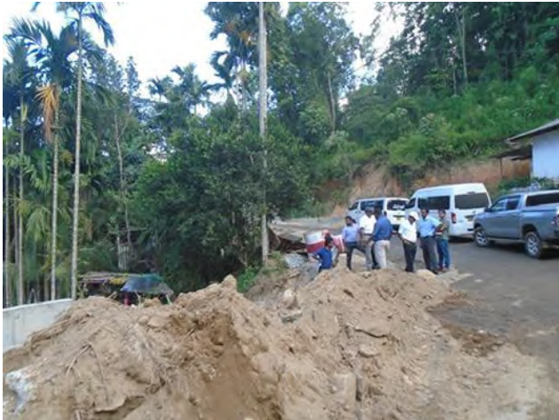
Figure 2-17: Field inspection to Badulla – Chenkalady (Bibila – Lunugala section) Road
