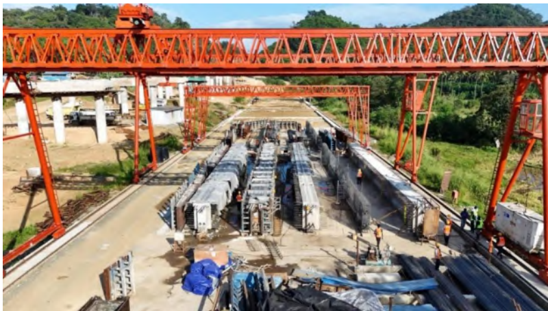
Figure 2-29: Civil work of the Central Expressway – Section III
