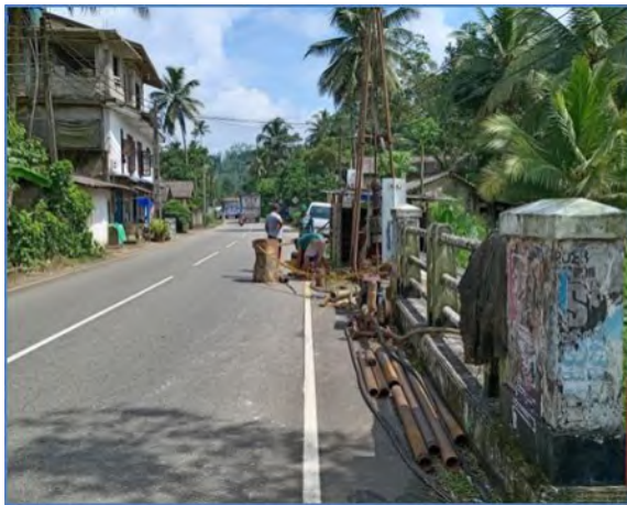
Figure 2-8: Borehole Investigation of Bridge. No- 22/5Km on Ambalangoda – Elpitiya –Pitigala Road
