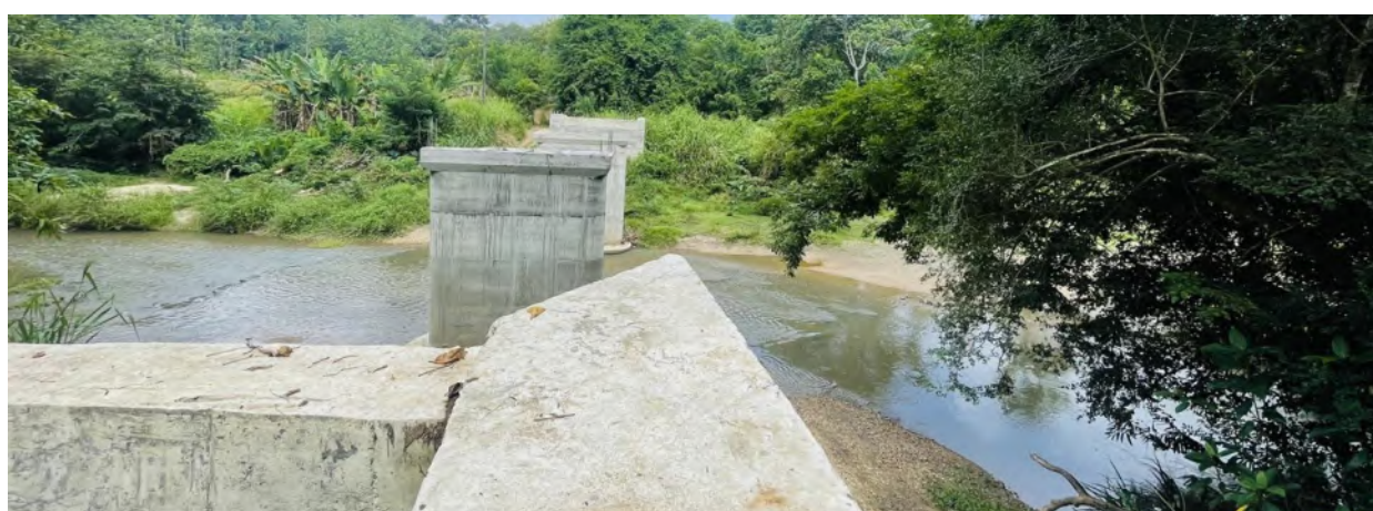
Figure 2-3: Construction of Bridge across Dahamal Oya on Kalugahawadiya Kehelkottuwa road in Bibile
