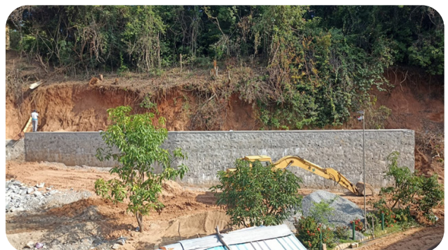
Landslide mitigation project at Hatthota Amuna, Matale
