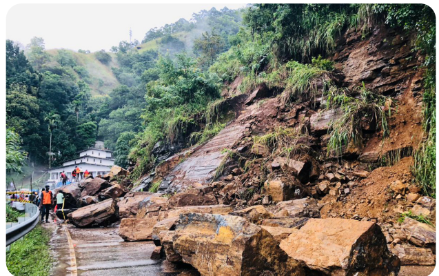
Landslide at Passara - Monaragala Road
