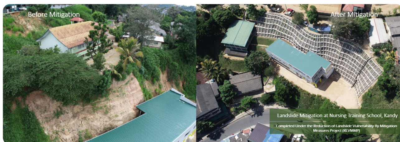
Landslide Mitigation Completed site - Nursing Training School Teaching Hospital, Kandy (Site No – 035 L2) – Package 05B
