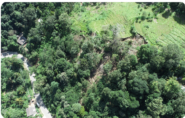
Landslide at Maliththagolla
