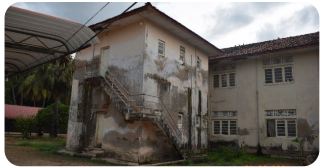
Nurses quarters building at Batticala teaching hospital
