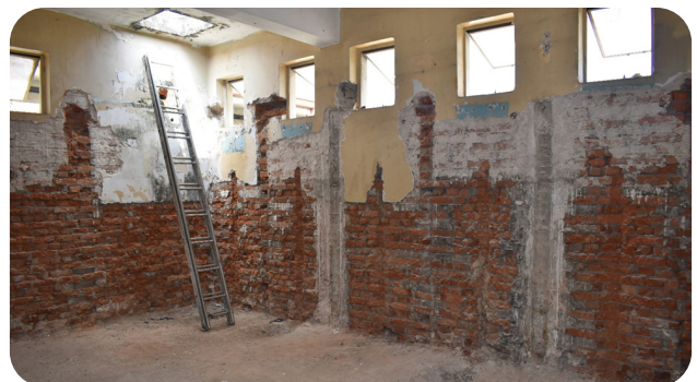
Renovation Project at Survey Department, Colombo 05
