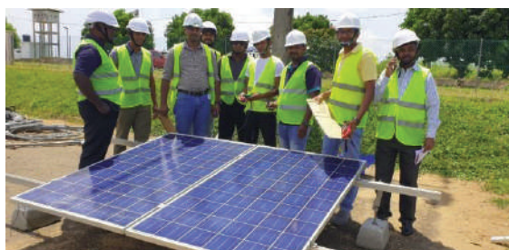
Figure 9: Rooftop Solar training programmes
