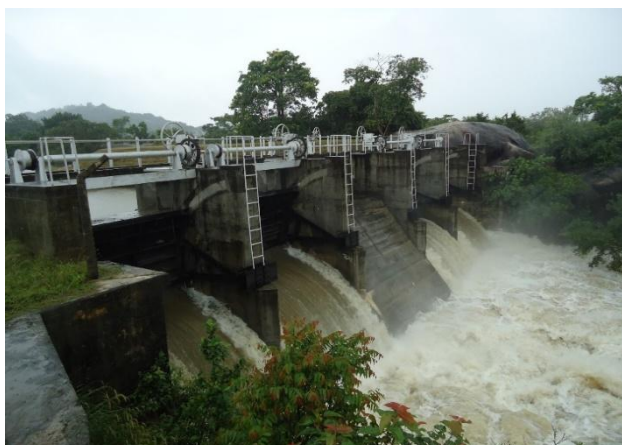
Water Gates of Pulugunavi Project
