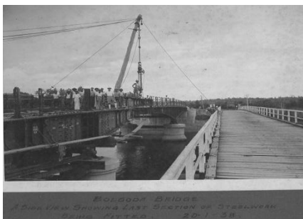
Bolgoda steel bridge –Side view
