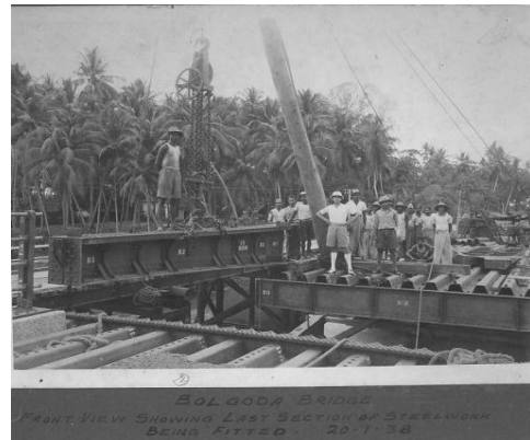
Bolgoda Bridge- Front View
