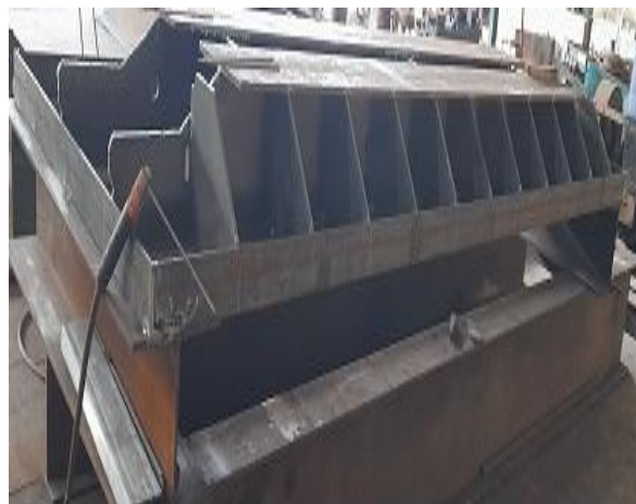
Fabricating gates for Oliyamulla
