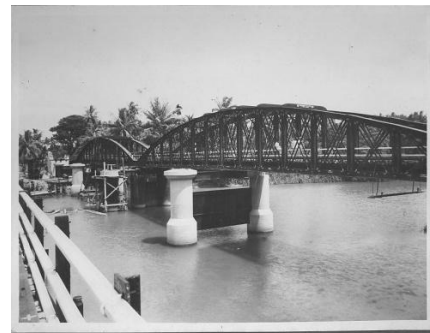
Thoppuwa Bridge 24 October 1938
