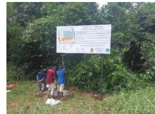
FIGURE 35 : INSTALLATION OF SIGN BOARDS
