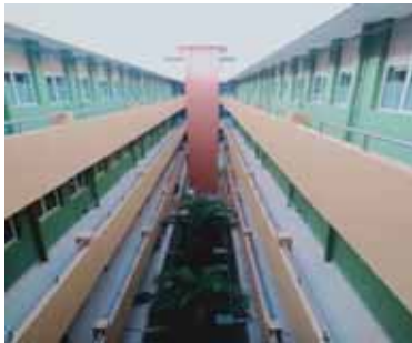
DGH Hambanthota - Isolation Building
