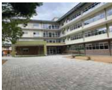
Base Hospital Mahiyanganaya
