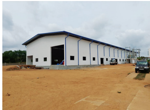
Figure 1 - Scrap Aluminium Recycling Plant
