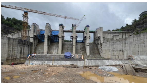
Dam under construction
