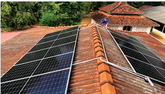
Installation of solar PV facility
