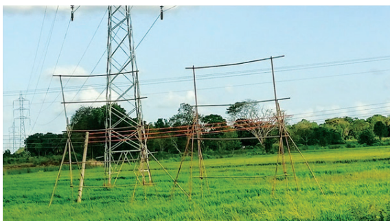
De-stringing works at section H107 – H115 in Package 4A , Anuradhapura- New Habarana Line
