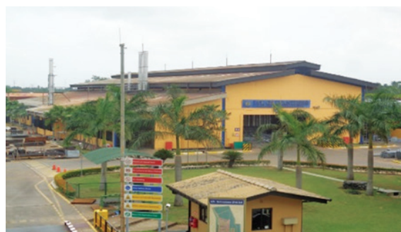
Galvanizing Plant at Sapugaskande
