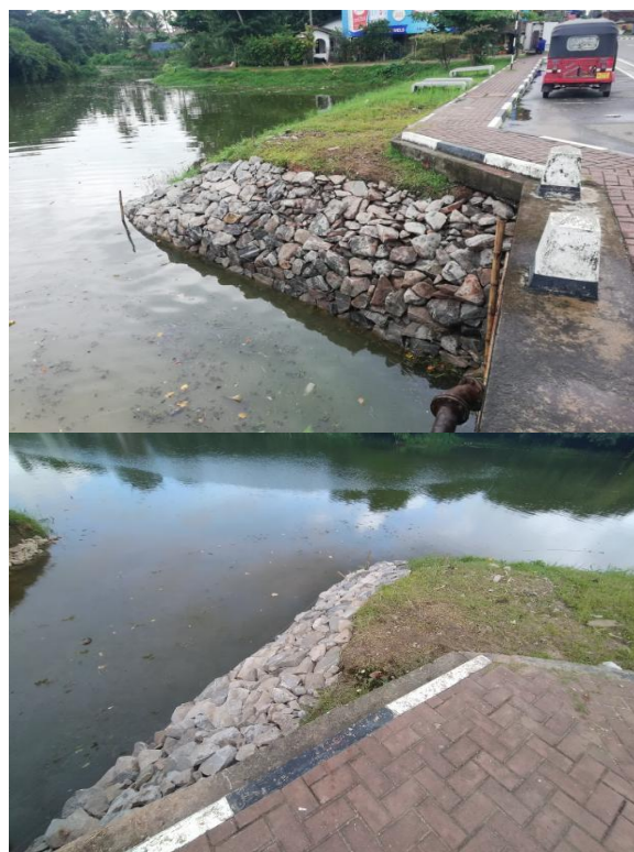
Rubble Packing on ITN Lake Banks at Drain outlet
