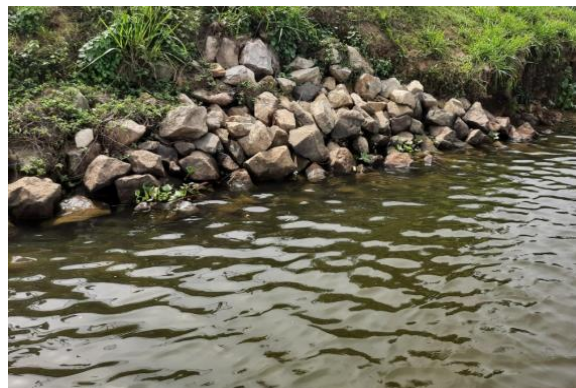
Rubble Packing on Embankment including Trimming and Forming of Slopes in Sea Plane Landing Bay at Diyatha Uyana
