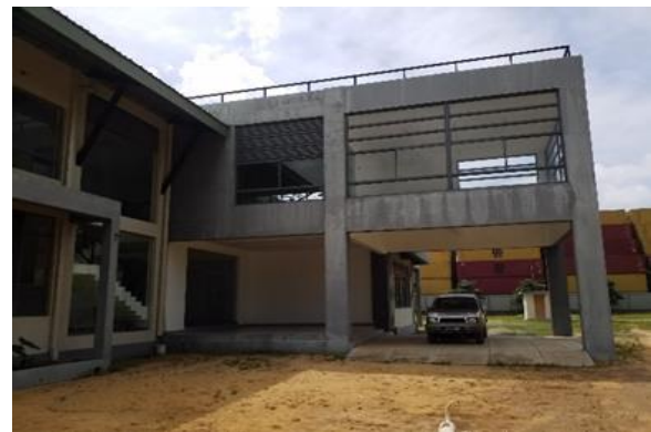
Figure13: Completed Workshop Facilitate Building
