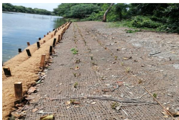
Figure 1: Just after finishing the restoration process
