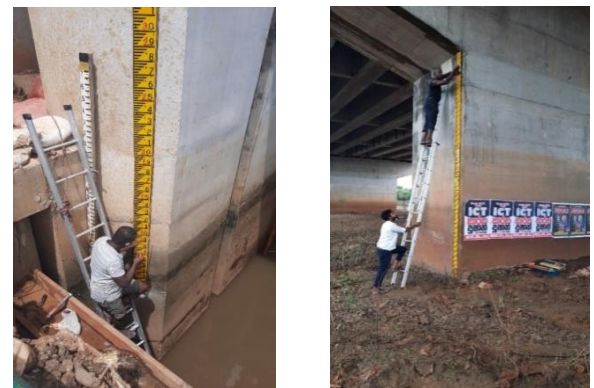
Figure 08: Installation of water level gauges
