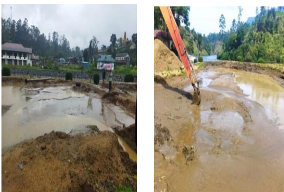
Figure 06: Progress of De- silting
