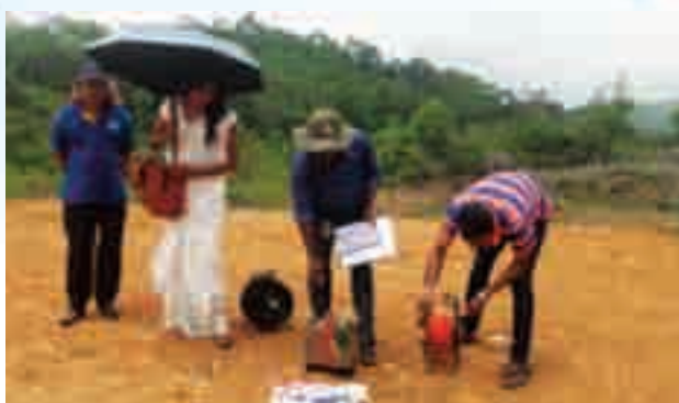
Figure 41: Groundwater investigations for soil excavation area
