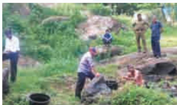
Figure 42: Monitoring of proposed rock excavation project area
