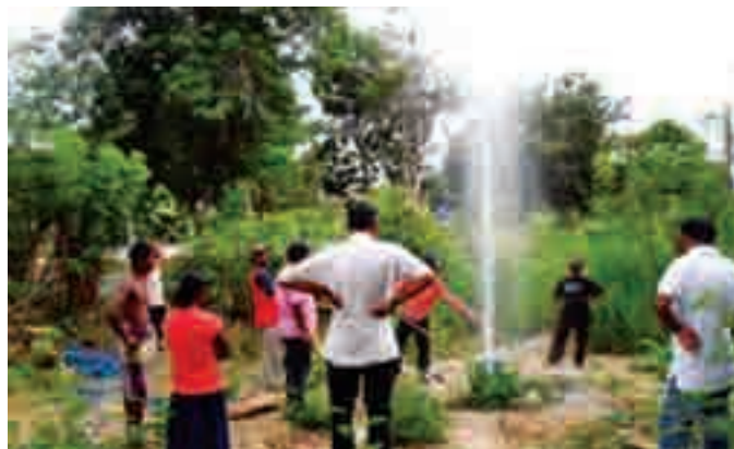
Figure 45: Tube well cleaning
