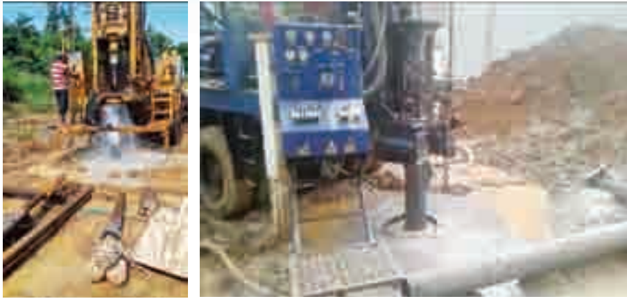
Figure 43: Tube well drilling
