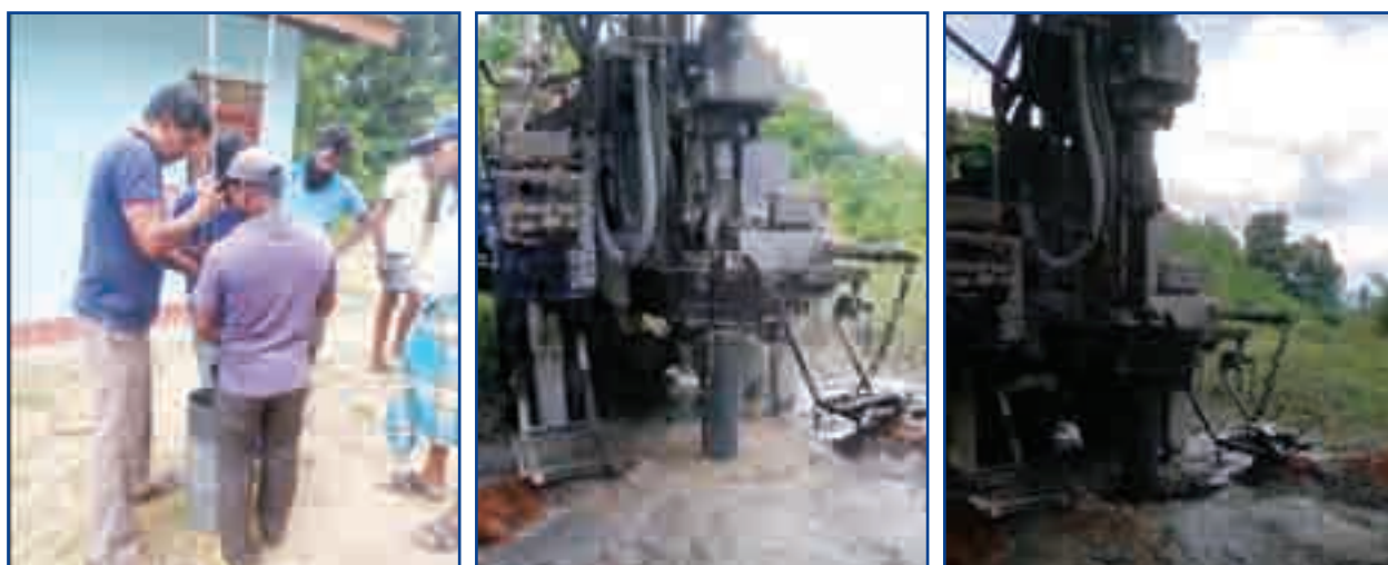
Figure 38: Tube well construction
