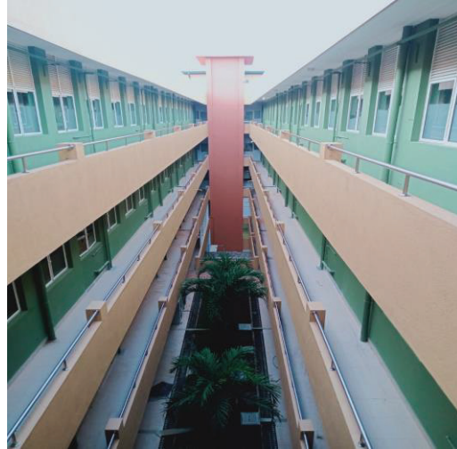
DGH Hambanthota - Isolation Building
