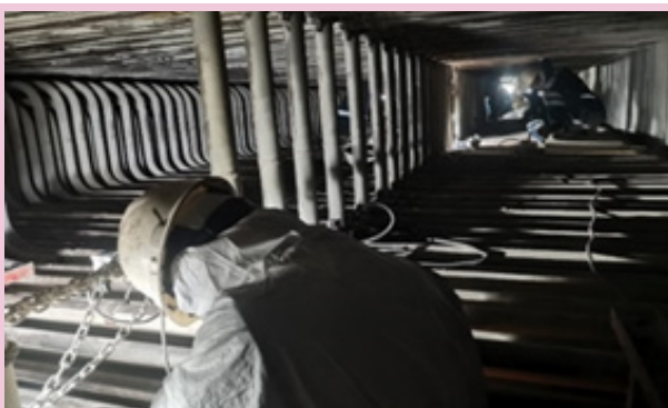
Figure G2: LTSH repair in progress
