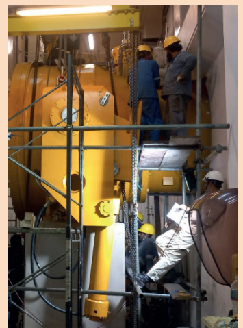
Figure G8: MIV repair in progress.
