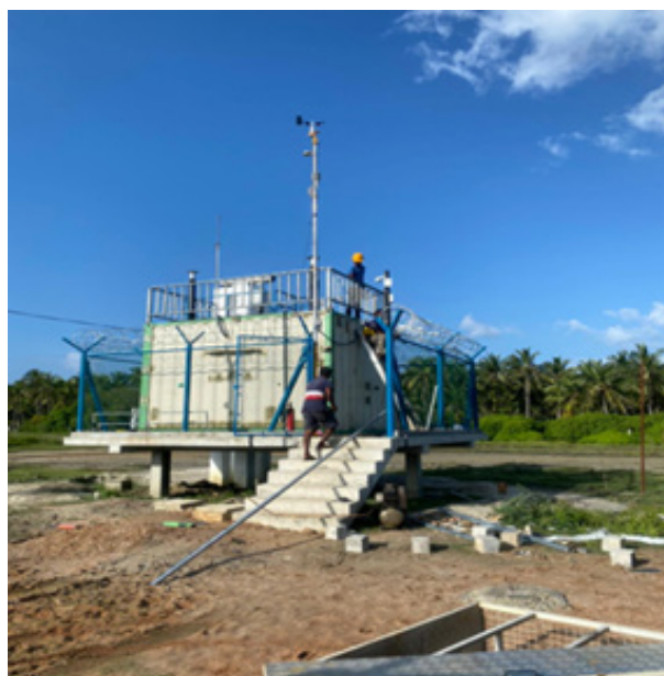
Figure S4: Ambient air quality monitoring station
