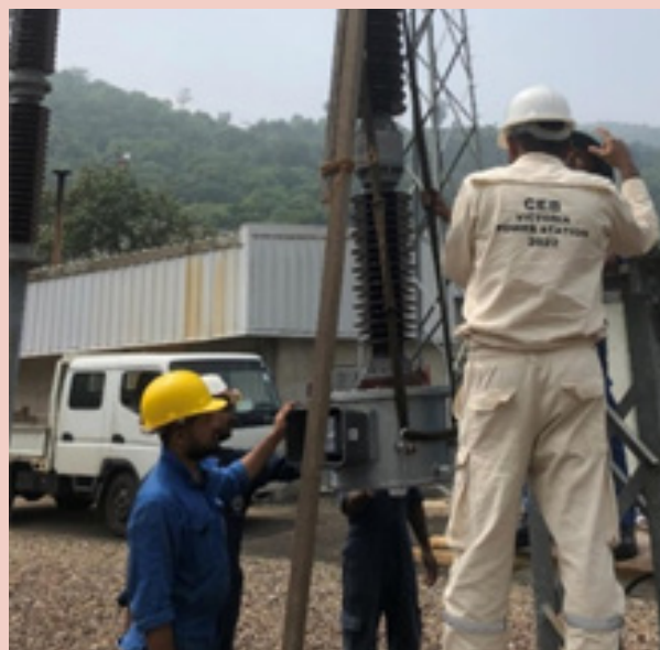
Figure G3: CVT installation in progress
