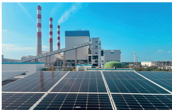
Figure C1: Rooftop solar PV system installed at LVPP.
