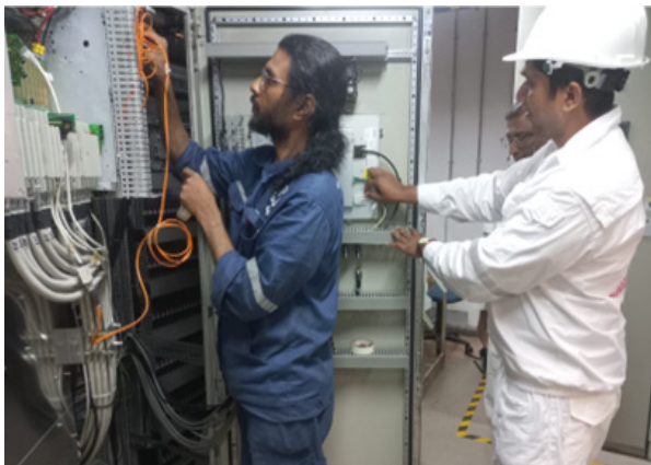
Figure G5: Installing and wiring of Controllers in progress.
