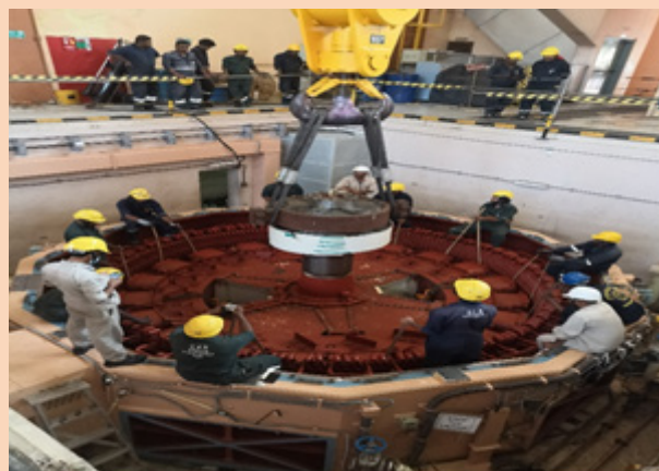
Figure G4: Turbine headcover replacement in progress
