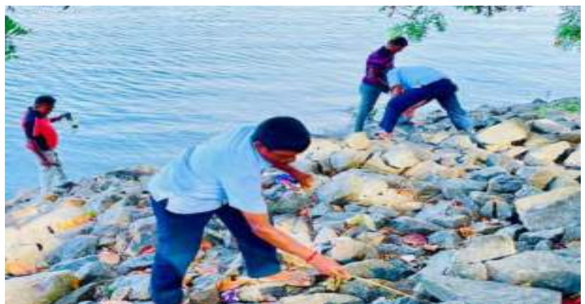
Figure 2.16: - Cleaning the embankment of Kala Wewa – Post Office, Negampaha.
