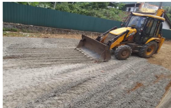
Fig 2.4 – Car Park – Modarawattha
