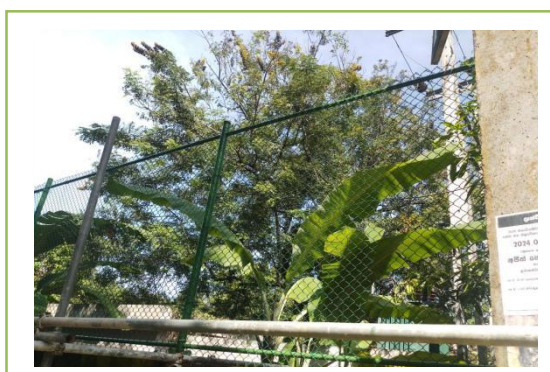
Fig 2.5 - Renovation of the Border Fence
