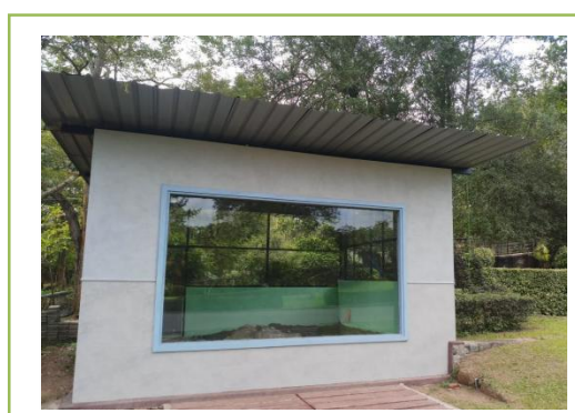
Fig 2.6 - Construction of Loris Enclosure
