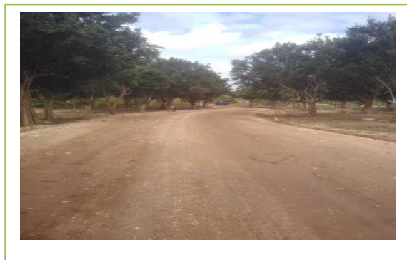
Fig 2.8 - Phase II Road Reconstruction in the Elephant Zone
