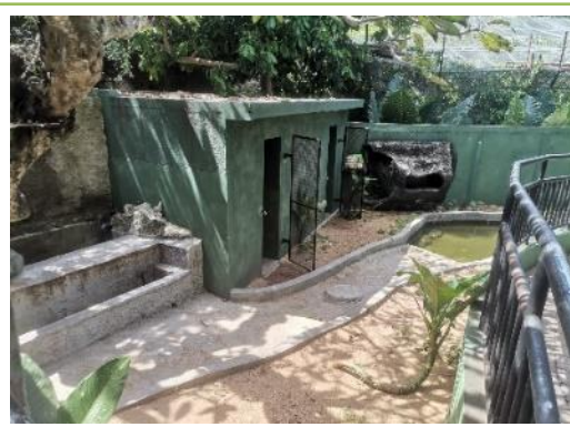
Fig 2.2 - Renovation of Animal Shelter – otter' Enclosure
