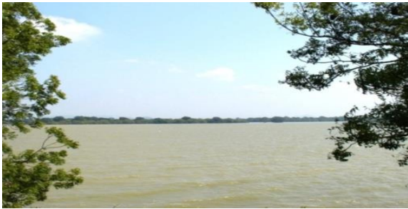
Kala wewa Reservoir Capacity: 123 million cubic meters
