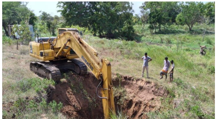
Digging Agri wells - 264
