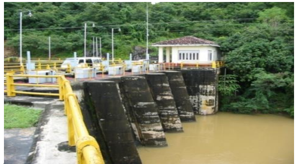
Minipe Reservoir Capacity: 0.12 million cubic meters
