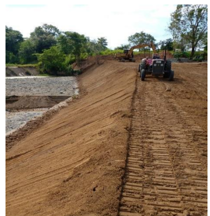
Repairing outer spill of Maldeniva Tank
