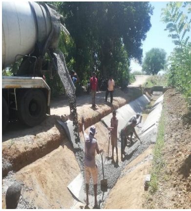
Wijepura 403/D12 Canal Repair
