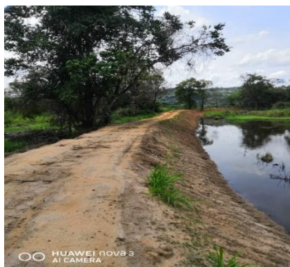
Constructing Miriswellanda tank
