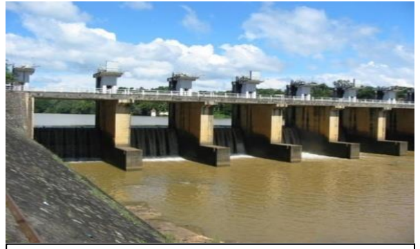
Polgolla Reservoir Capacity: 4.1 million cubic meters
