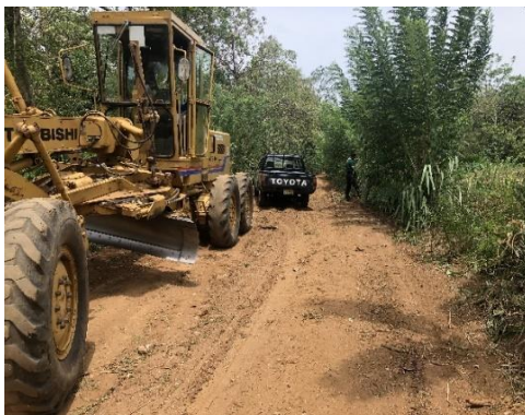
Constructing roads using motor graders
