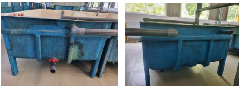
Figure 1: Existing facility before modification
