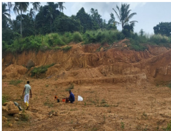
Figure 33: Groundwater investigations for soil excavation area
