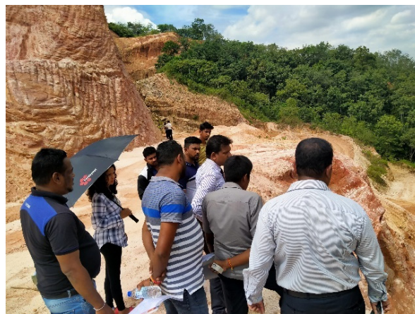
Figure 27: Join inspection at Madabawita soil excavation site
