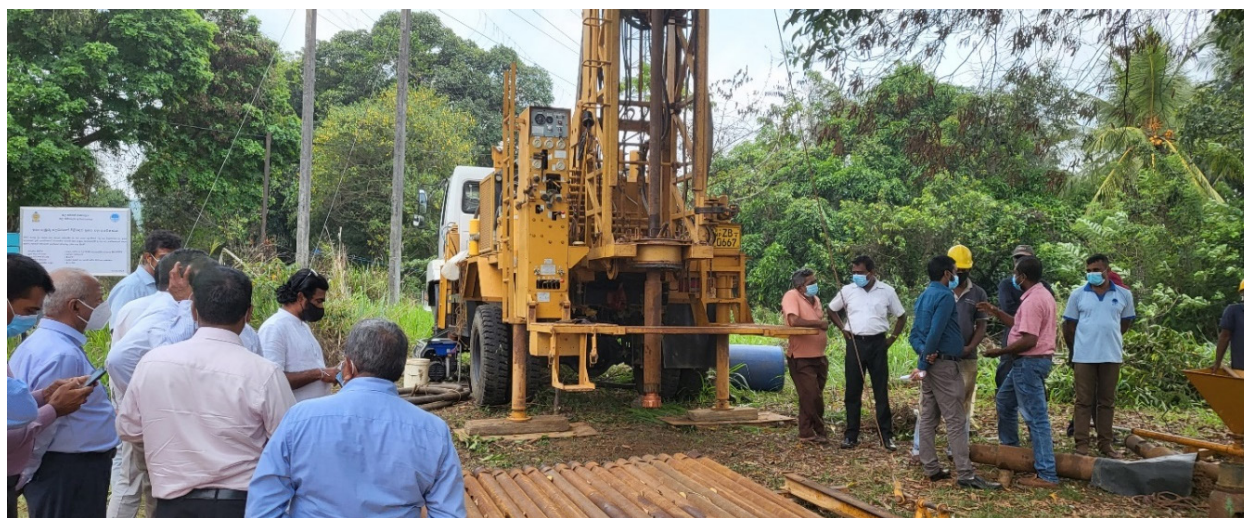
Figure 25: Initiating the drilling of deep borehole in Alawwa Pallemorugama area
