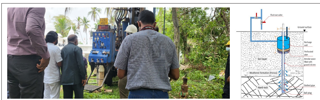
Figure 22: Initiating the drilling of deep recharge well at Bemmulla Sri Wardhana Pirivena and the proposed recharge structure diagram.
