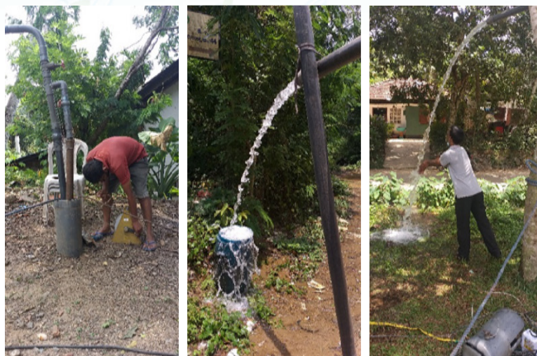
Figure 31: Conducting pumping tests in Matara area
