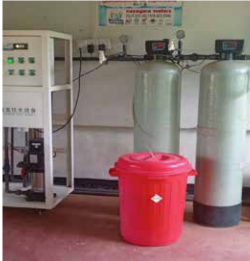
Water Purification Machine repaired in the Galnewa War Hero Village
