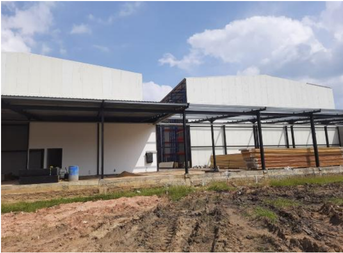
Constructions works of the stores complex are in process
