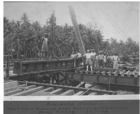
Bolgoda Bridge- Front View
