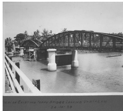
Thoppuwa Bridge 24 October 1938
