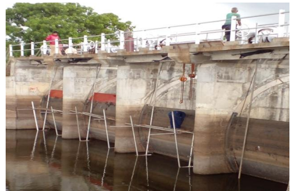
Renovations at Kanganikulam
