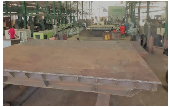
Fabricating gates for Oliyamulla
