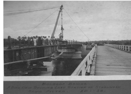
Bolgoda steel bridge –Side view
