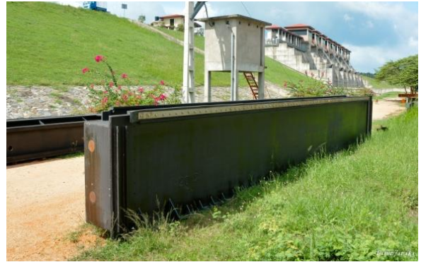
Deduru oua project emergency Water control gate
