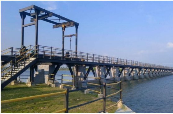
Water control gates at Thondamanaru barrage
