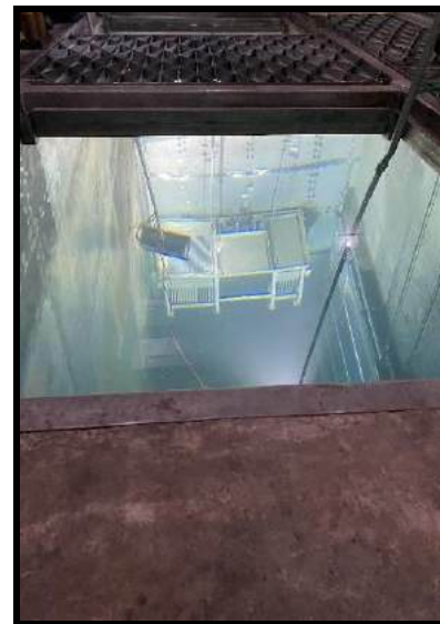
Fixing Co-60 pencils in the source rack
