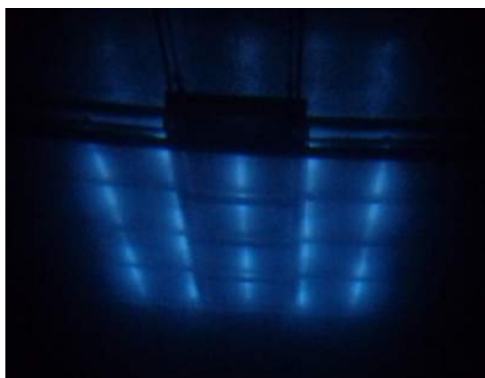
Co-60 pencils (30 nos.) in the water pool, before source upgrade
