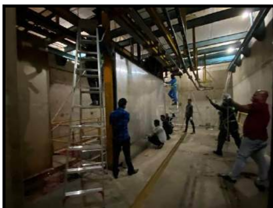
Dismantling heavy structures in the source chamber
