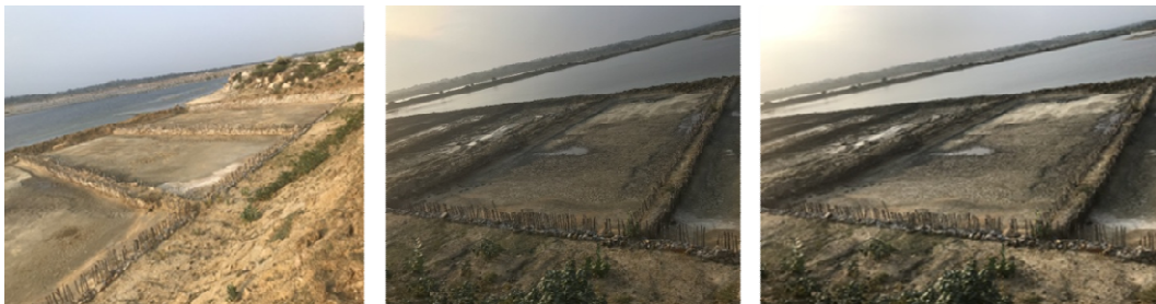
Figure 1, 2 and 3: Partially constructed three ponds at Hambanthota
