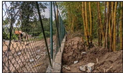
Renovated boundary fence at GMPG
