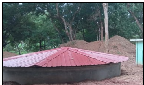
Constructed Agro well at MTC
