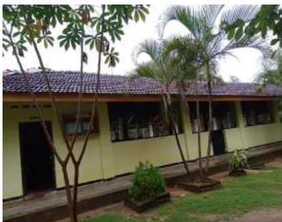
Renovation of the Dharmashala Building of Manabharana Viharaya Siyambalanduwa
