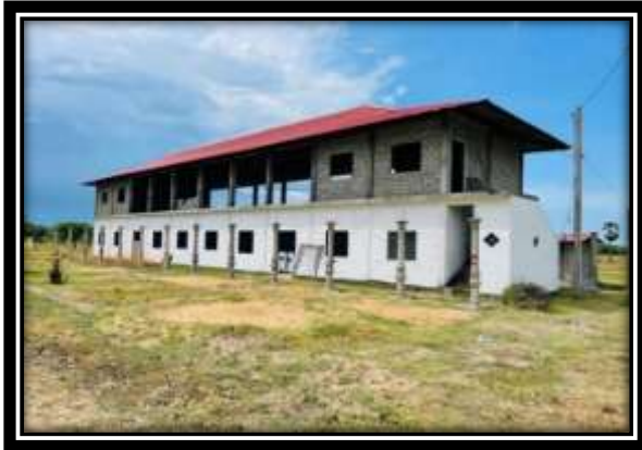
Completion of Daham School building at Welgam rajamaha viharaya in Trincomalee
