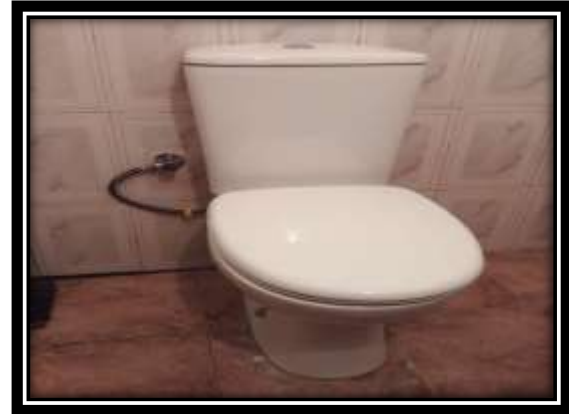
Construction of Common toilet complex in Thissa Rajamaha Viharaya
