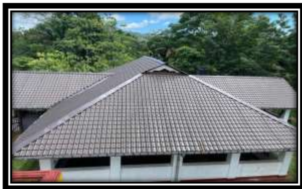
Completion of Dharmashala Building at Delgamuwa Rajamaha Viharaya Ratnapura
