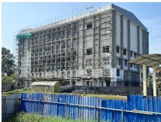
Figure 6.8: Multi-Purpose Building, Wayamba University of Sri Lanka, Makandura Premisses
