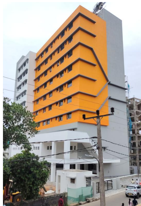
Figure 6.9: Project of constructing a 12 storied building for the Faculty of Medicine, University of Ruhuna
