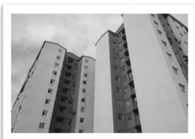
Kolonnawa Housing Project
