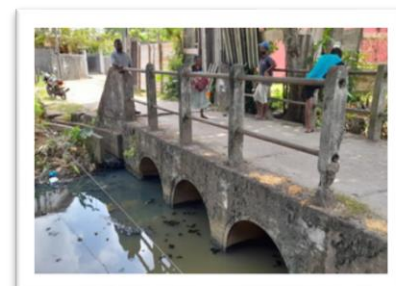
Construction of Dhammawela canal - Wennawatta road culvert
