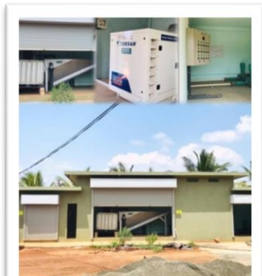
Construction of Sewer Treatment Plant (Capacity - 75m 3 /day)
