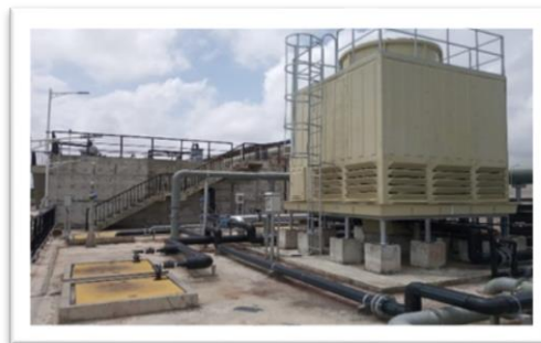
Leachate Treatment Plant
