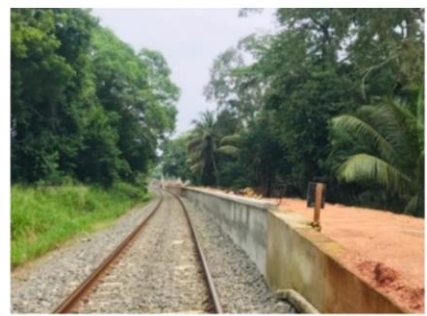
Construction of Railway Platform (Length - 318 m)
