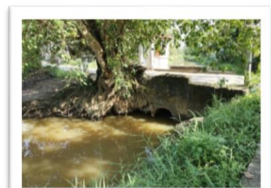
Construction of Selalihini Mawatha canal
