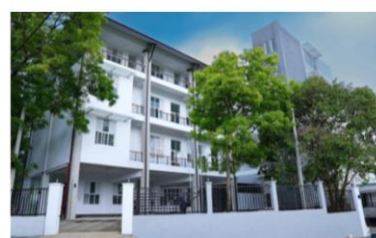
Construction of Courts Complex, Theldeniya (TEC - 599 Mn.)
