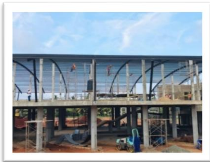
Construction of Two storied Bus
