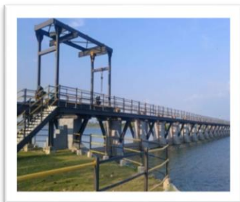
Water control gates at Thondamanaru barrage
