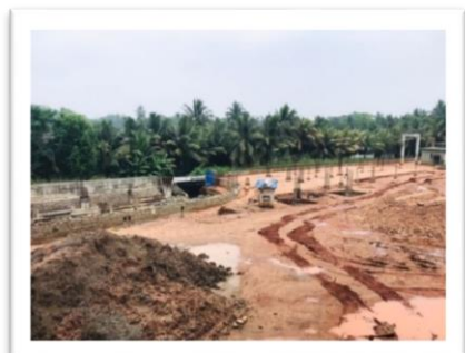
Construction of Two Storied Railway
