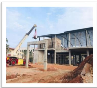
Construction of Overhead Bridge (Connection of Railway Building to Bus Terminal Building)
