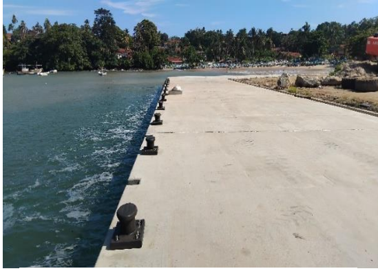
Construction of the quay wall
