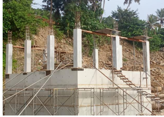
Underground water sump
