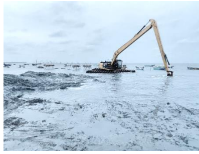
Cleaning the canal
