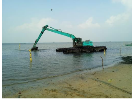
Cleaning of the Existing Access Poonakary
