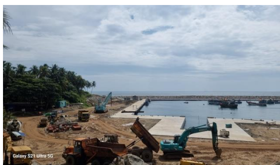
Construction of travel lift bay
