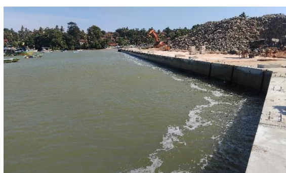
Construction of the quay wall
