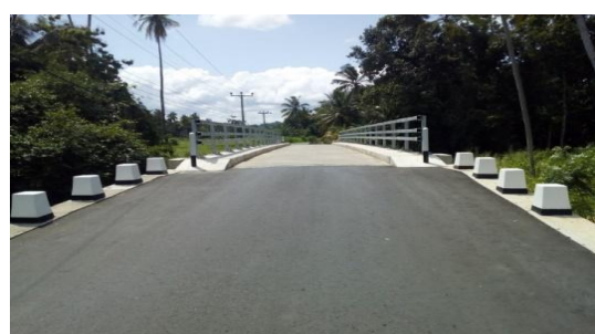
Bridge No. 5127, Kurunagala Kosdanda Canal Bridge
