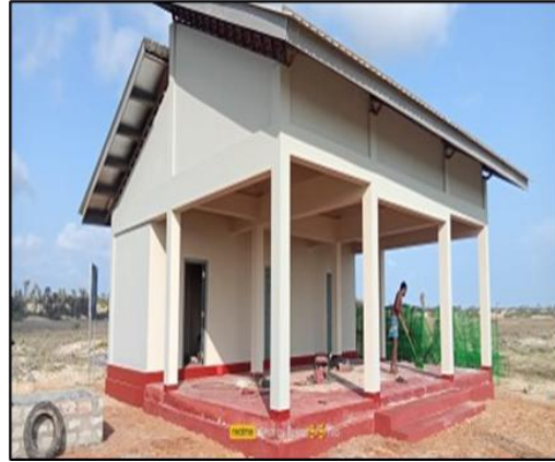
Construction of Tourist service centre with sanitary facilities at Casurina Beach
