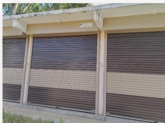
Construction of stalls for the Karametiya weekly fair Meegahakiwula P.S. Uva Province
