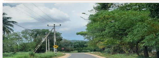
After improvement of Himbutugollewa – Thammannagama – Kolongaswewa Road in Galenbindunuwewa Divisional Secretariat of Anuradhapura District
