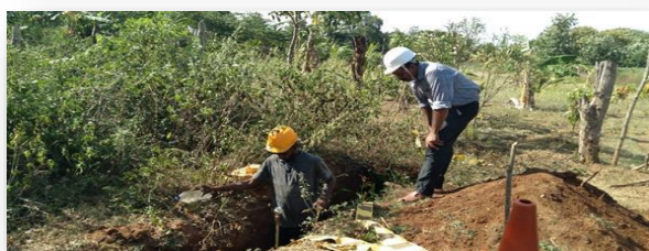
Pipe laying works at Puthiavellar Sinnakulam Drinking Water Project, Vavuniya South Tamil
