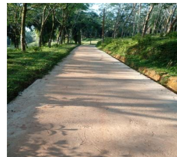
Concreted the Dodangoda Talemulla road RS.Mn. 3.0
