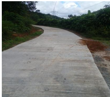
Concreted Dodangoda Wasanhena road Rs Mn. 4.0 (In front of the Eladuwa primary tamil college)
