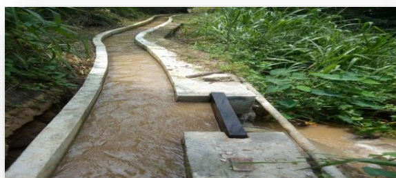
Rehabilitation of Mahantewela Anicut and Canal in Kandekatiya PS Area of Badulla District
