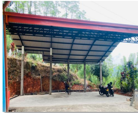
Repairing the Kalawana Pradeshiya Sabha Office building and the vehicle park Kalawana P.S. – Sabaragamuwa Province
