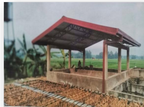
Construction of Gully Waster Treatment Center in the Pannala Pradershoya Sabha
