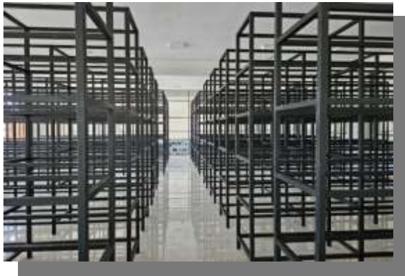
Internal partitions, fixing of racks in the Land Registry Batticaloa
