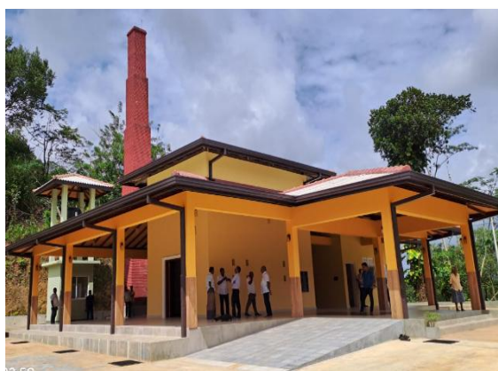
Construction of crematorium building and external work of Neluwa Pradeshiya Sabha Neluwa P.S. Southern Province
