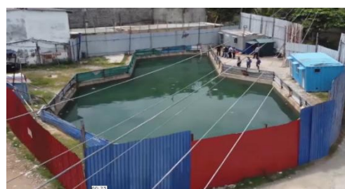
Thalakotuwa Garden Pumping Station
