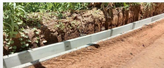
Construction of U type side drains on Welanhinna - Kirigalpotta road in
