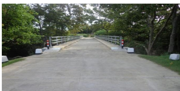
Bridge No. 5115, Thellulla Bridge over Monaragala Kirindi Ova
