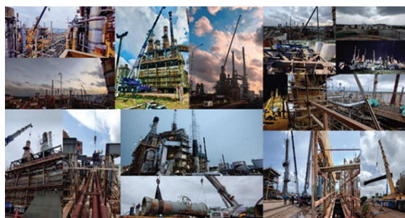
(Renovations at Refinery)
