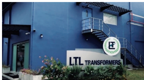
(Transformer Plant at Angulana)
