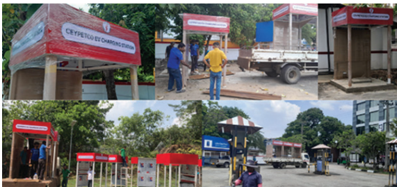
(Electricity Vehicle charging Points)
