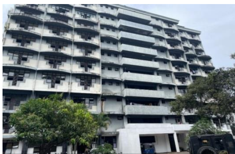
Construction of Kuruduwatta
