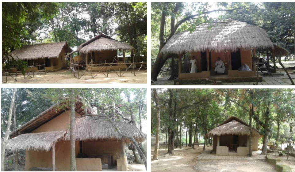
Renovation of existing village houses in the “Ape Gama” premises and installation of Cogon grass roofing
