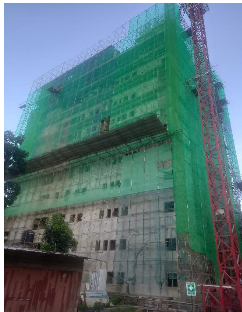
Figure 6.8: Project of constructing a 12 Storied Building for the Faculty of Medicine, University of Ruhuna
