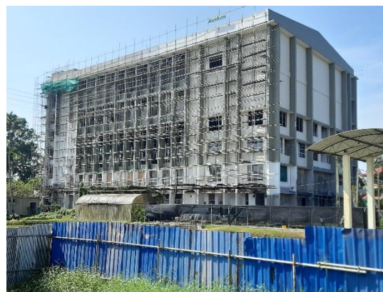
Figure 6.5: Multi Purpose Building, Wayamba University – Makandura Premises
