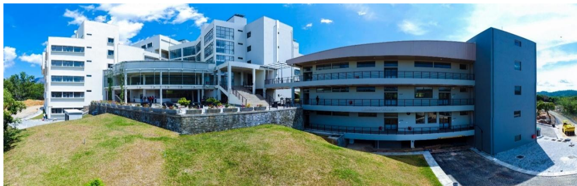
Figure 6.2: Design and construction of buildings and infrastructure for the Faculty of Computing and Technology, University of Kelaniya
