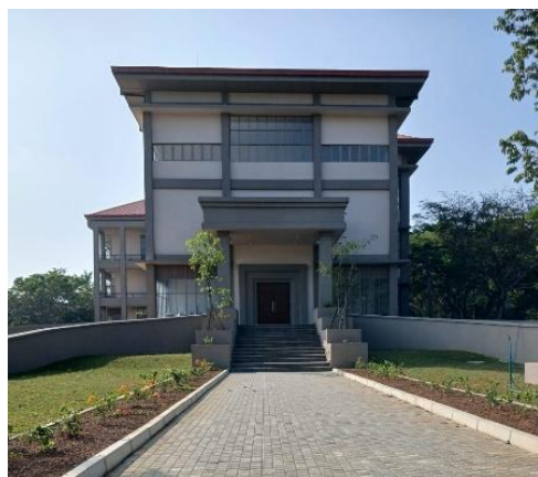
Figure 6.4: Library Building, Wayamba University – Kuliyaipitiya Premises
