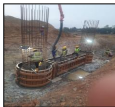
Concrete pouring for the Tie beam at VD 09 (16+523-17+986) at VD 08 (15+288-16+188)
