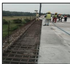
Concrete pouring for the balance section of the 100mm deck slab at VD 08 (15+288-16+188)
