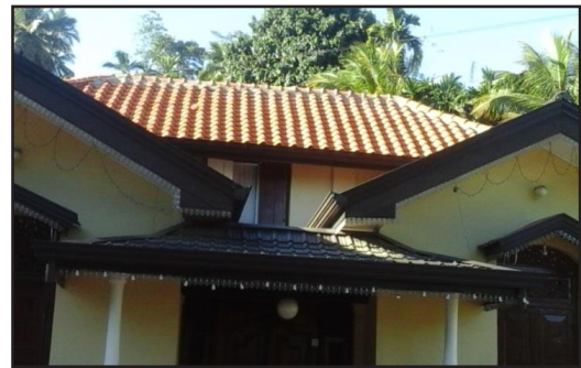
Renovation of roof Asgiri Gunnepana temple - Rs. 590,000/
