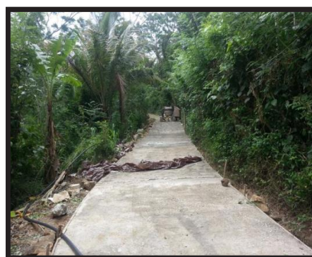
Concreting of Waligepola Makulgahamada Road Rs. 0.23 Mn
