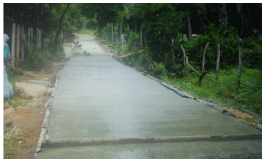
Concreting of Wellaimannal Neroththumunai 5 th Lane in Trincomalee Rs. 1.5 Mn
