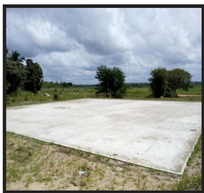
Constructing of thrashing floor at 242 in Dibulagala, Polonnaruwa Rs. 1.0 Mn
