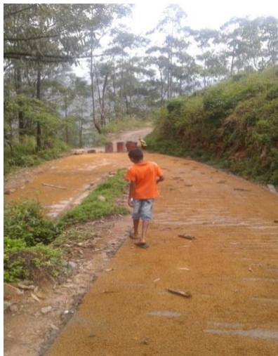
Concreting of Kirigala Karamatiya Road in Badulla Rs. 1.5 Mn.
