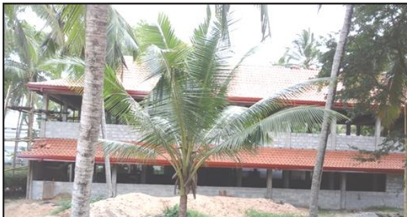
Making a roof for Dhamma School building in Jayasumanarama Temple at Mahava secretarial Division -Rs.300,000.00
