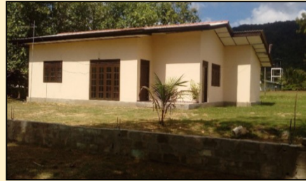
Buttala camp of Govt. Gazetted officers after completion
