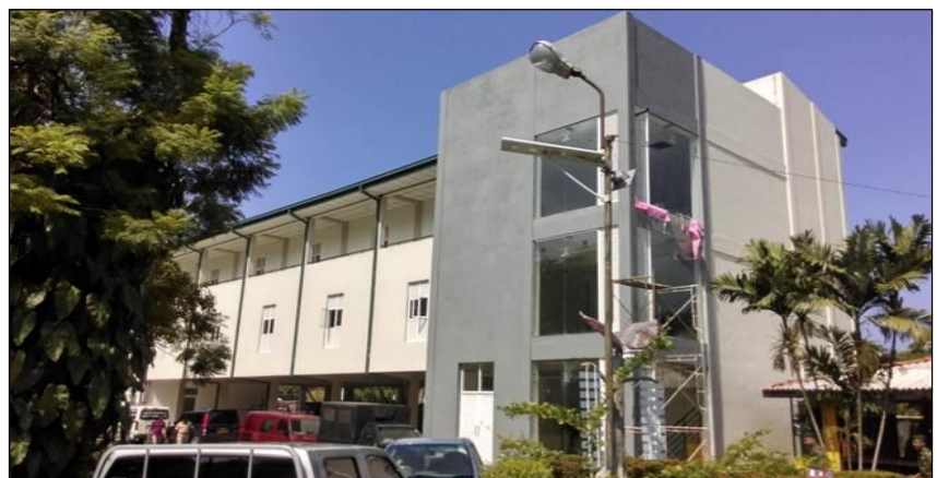
Office Building of the STF Headquarters being Constructed
