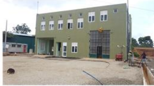
Puttalama Treatment Plant
