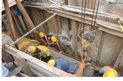
Un-expected underground utilities during the construction
